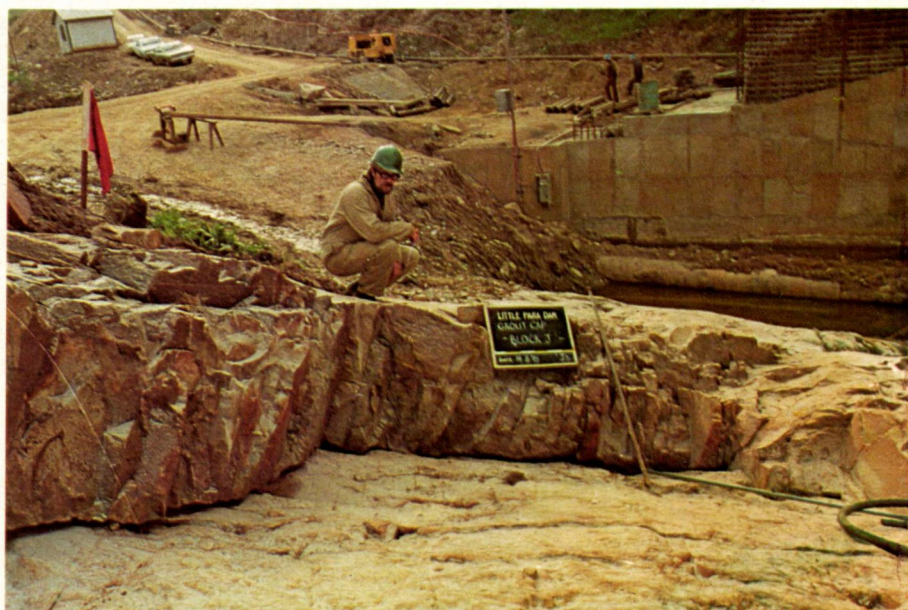
Plate 8 Left bank grout cap excavation—March, 1974 (T24376). 1. Hillside stress relief fracture. 2. Dental concrete in excavation seam of weathered dolomitic siltstone (Unit 13). 3. Shows slabby nature of dolomitic siltstone.
