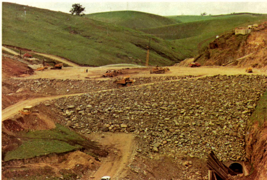
Plate 7 Upstream view of wetting and compaction of zone 3 rockfill in July, 1976 (T24375).
