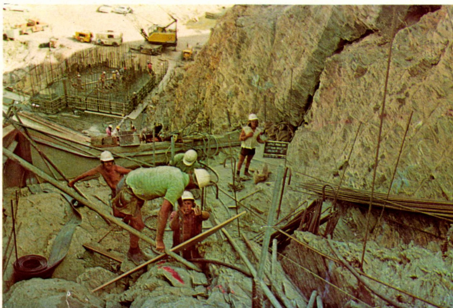
Plate 7 Upstream view of wetting and compaction of zone 3 rockfill in July, 1976 (T24375).
